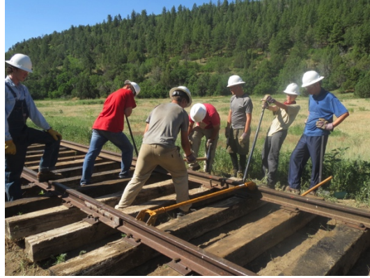
Laying railroad track at Metcalf Station
