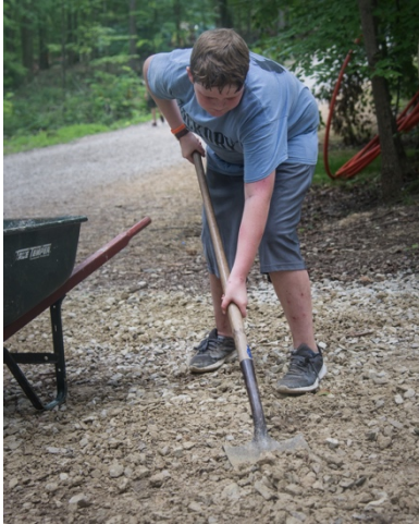
Charles Pelz working on a service project at Eagle Quest
