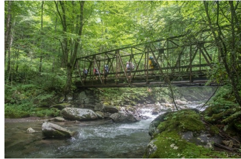
Crossing Bradley Fork Creek
