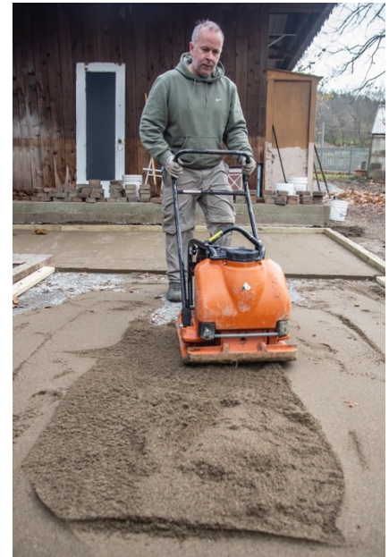
Mr. McGrath running the compactor
