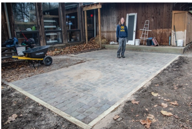
Isaac Lohmueller with the finished project
