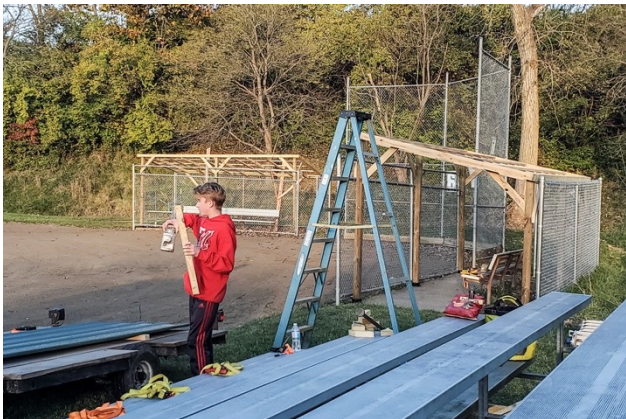
Wooden frames have been added to support the new metal roofing
