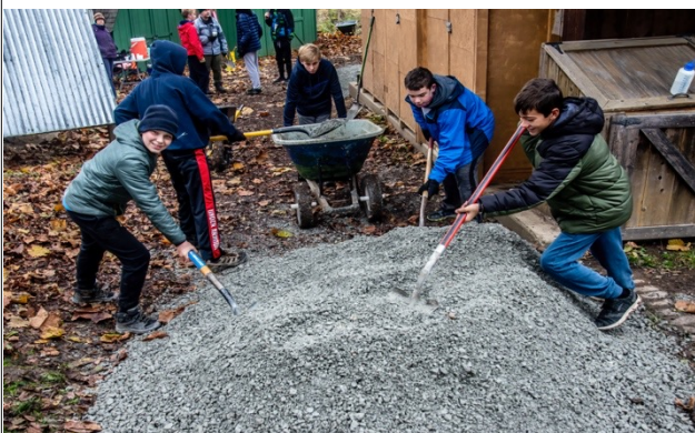
Moving gravel from the pile to the patio
