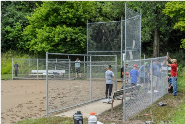
View of the field as the fencing work is underway
