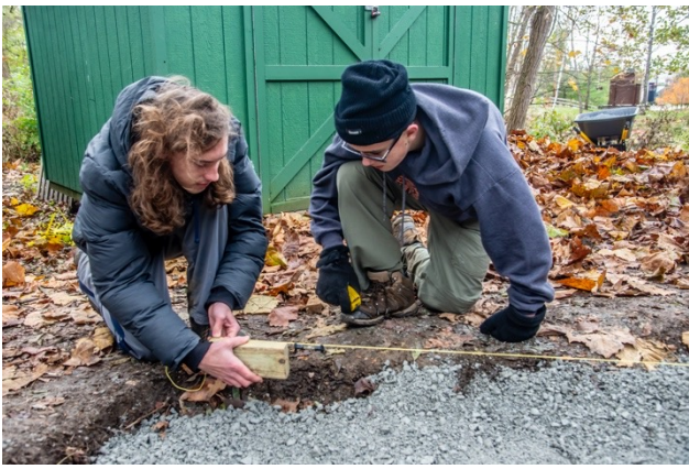
Isaac Lohmueller, Wesley Anglin checking the height of the gravel
