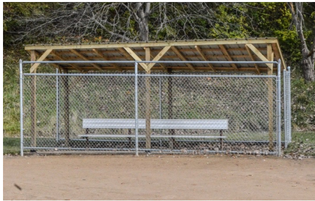
Finished first base dugout
