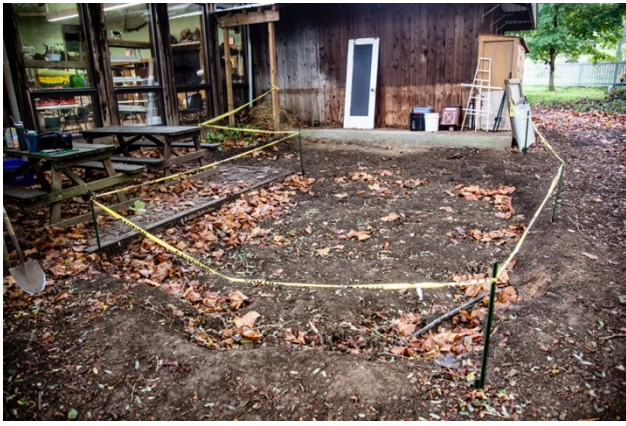
Between work sessions, Isaac roped off the work site
