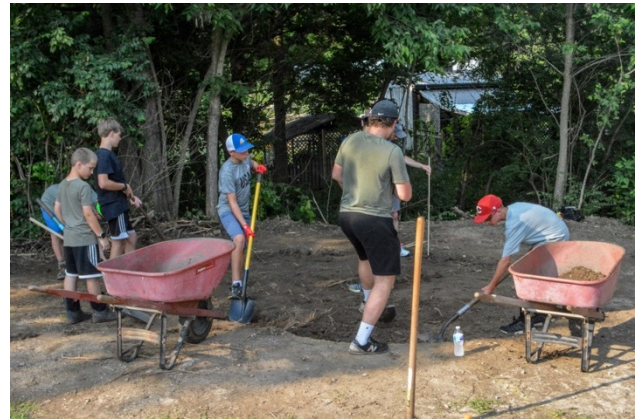
Digging a level foundation
