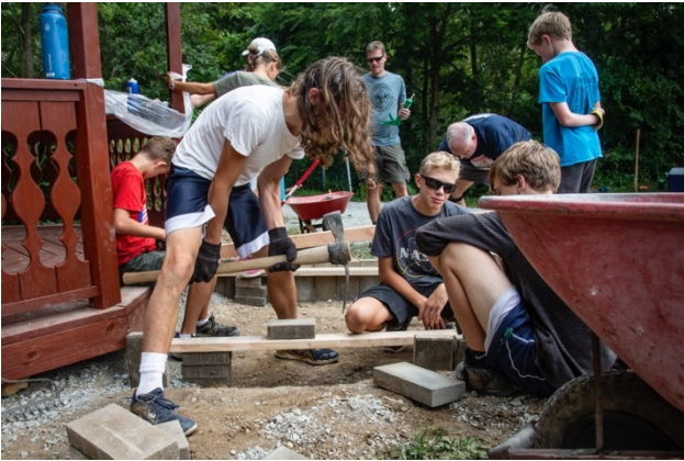
Laying the edging paver stones along the side of the walkway
