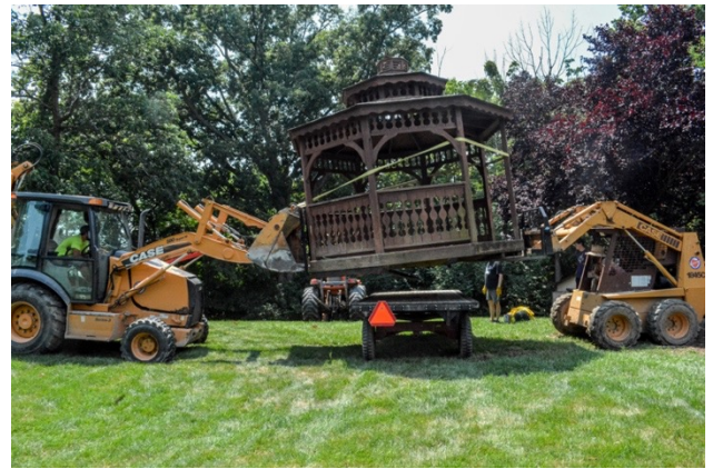
Placing the gazebo onto the trailer
