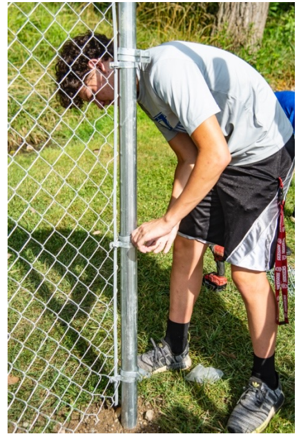
Nick Stroh securing the fencing
