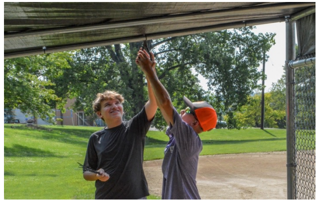
Nathan Hoffman, Declan McGrath securing the roof tarp
