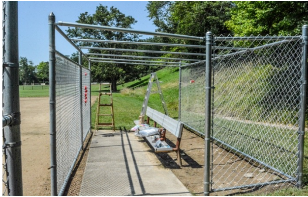
Roof bars have been added to the first base dugout
