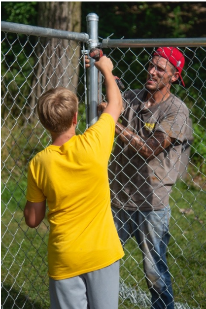
Ben Adkins tightening the fence strapping
