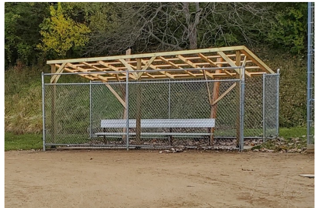
Completed wooden frame for the first base dugout
