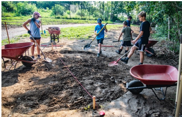
Digging out the foundation
