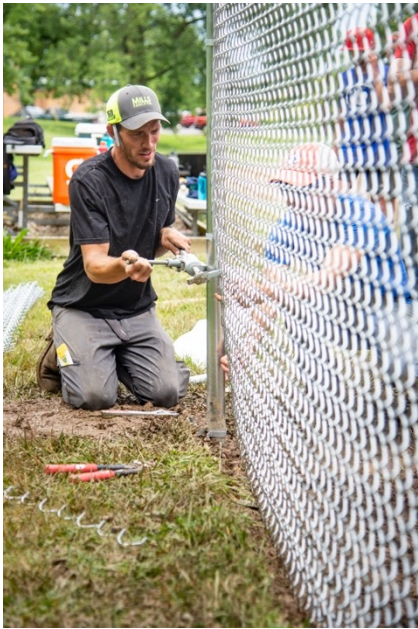
Declan McGrath benefited from the help of professional fence installer
