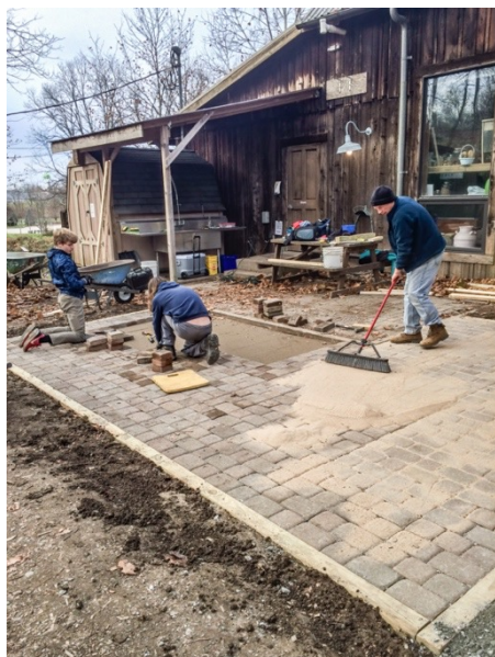
Mr. Lohmueller spreading the paver sand
