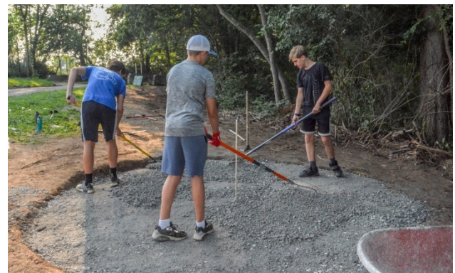
Spreading the gravel to form the foundation
