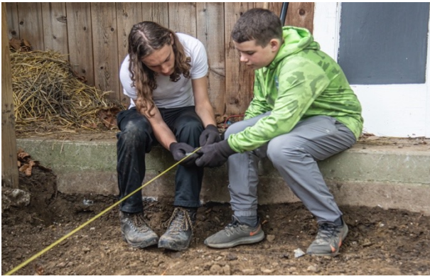
Isaac Lohmueller and Travis Anglin checking the depth of the foundation
