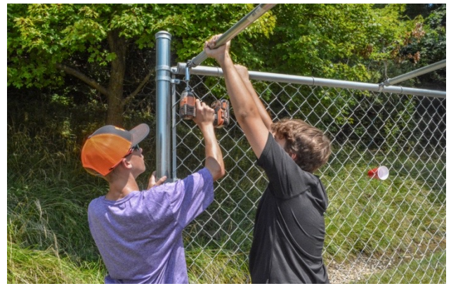
Declan McGrath, Nathan Hoffman installing the roof rails
