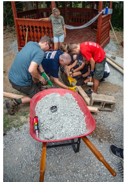
Laying down the edging paver stones
