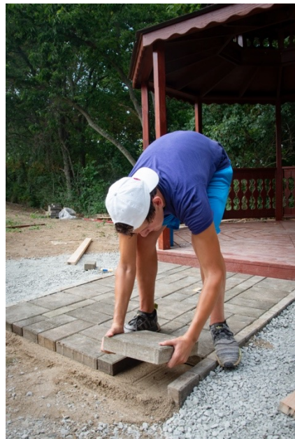
Nick Stroh placing the last paver stone
