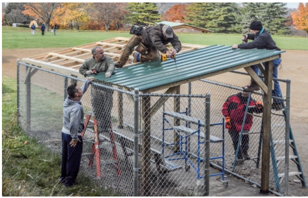
Installing the metal roofing
