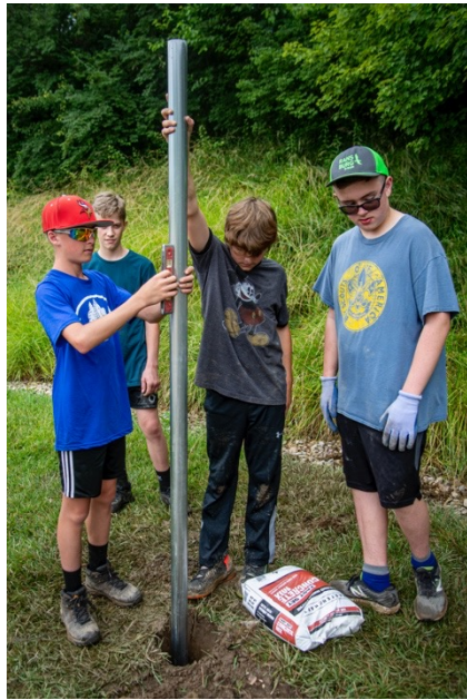
Setting the post for the fencing
