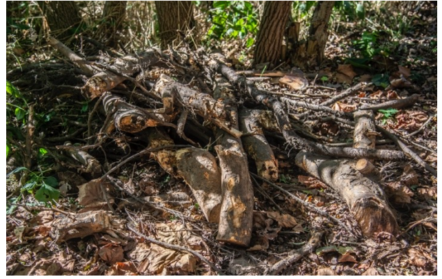
Big pile of roots removed from the work site
