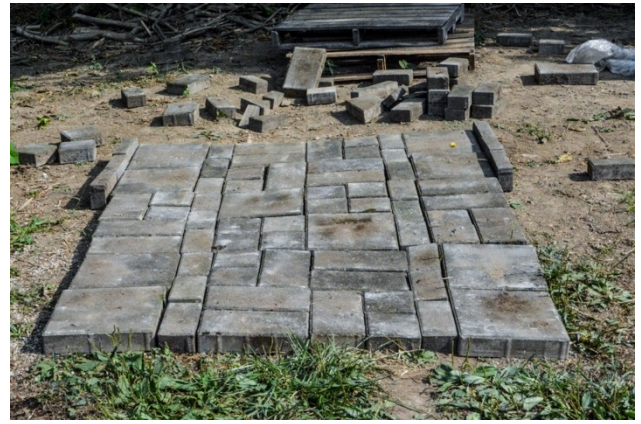
The final paver stone pattern
