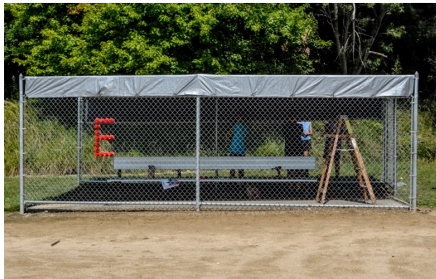
First base side dugout is complete
