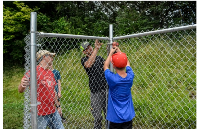
Declan McGrath tightening the fencing straps
