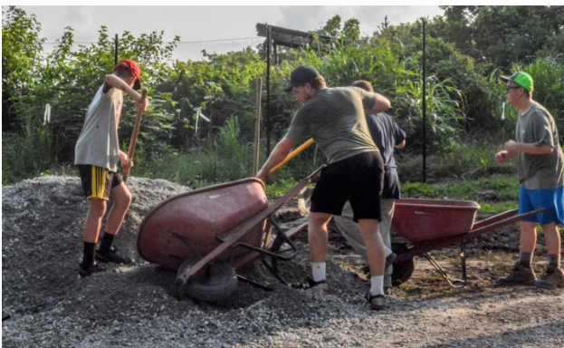
Getting wheelbarrow loads of gravel
