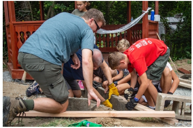
Laying the edging paver stones
