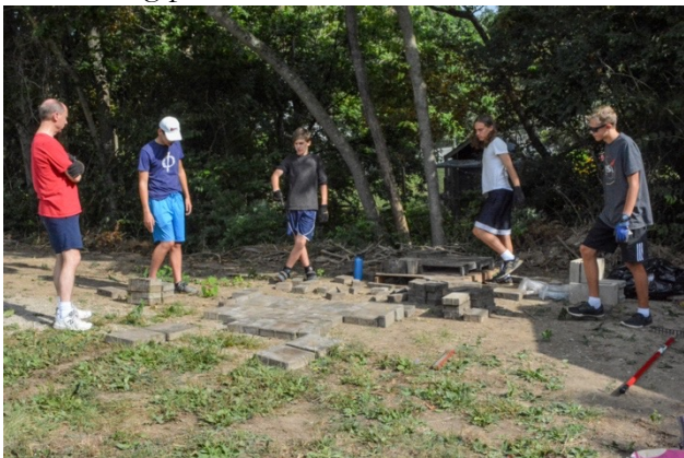
Discussing how to lay out the paver stone pattern
