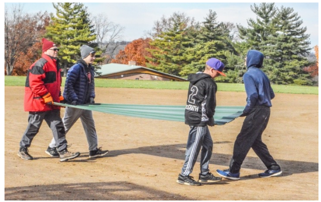
Mr. Wilkens, Petey Wilkens, Declan McGrath, and Isaac Lohmueller carrying a piece of the metal roofing
