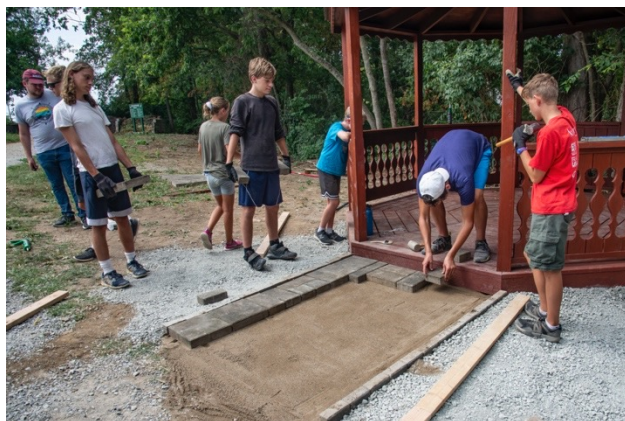
Laying the paver stones
