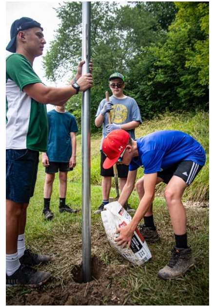
Setting the post for the fencing
