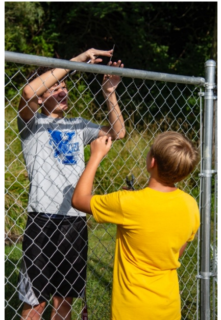
Nick Stroh and Ben Adkins attaching the fencing to the railing
