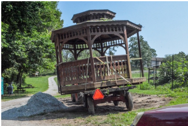
The gazebo was delivered to the work site
