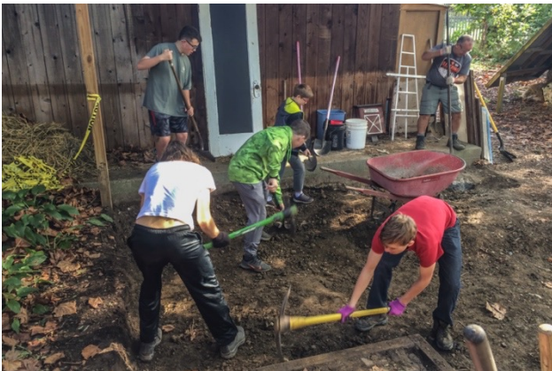
The Scouts had to dig down to get a flat foundation
