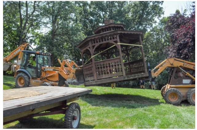
Using both the front loader and the bobcat loader, the farm was able to move the gazebo
