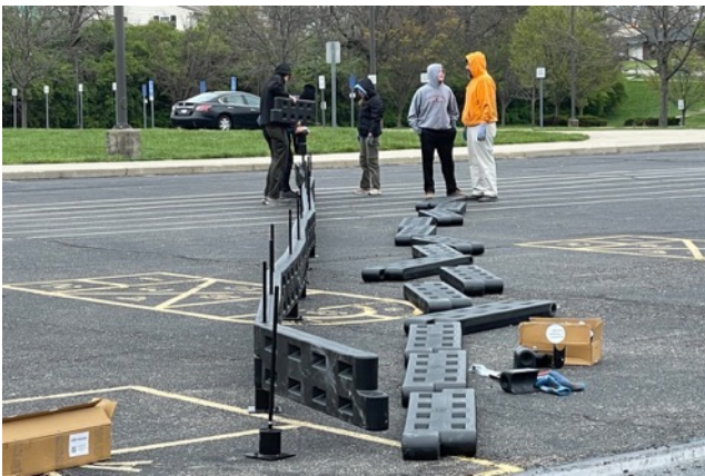
The next step was to build the wall around the pit
