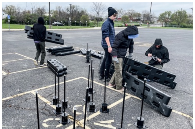
Assembling the wall
