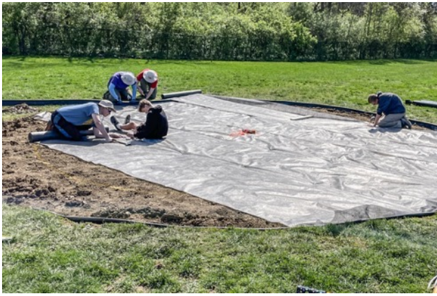
Laying the landscape fabric
