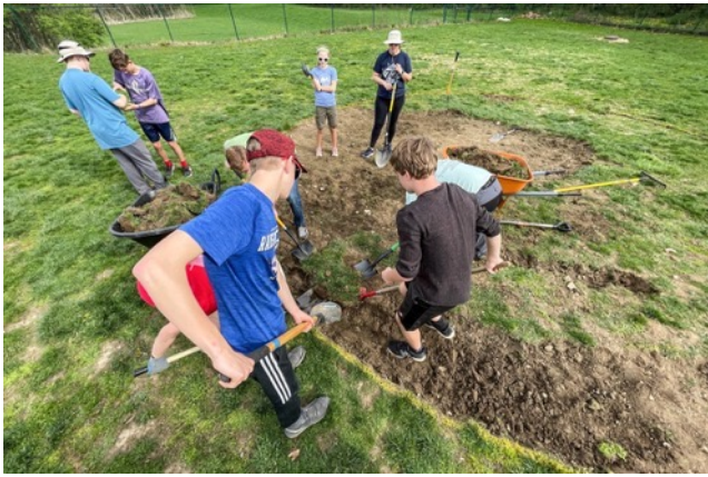
The scouts had to remove several inches of sod and dirt for the foundation of the Gaga ball pit
