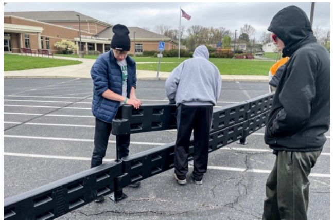
Petey Wilkens and Travis Anglin assembling the wall
