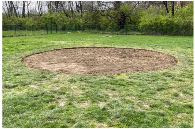
The finished base, ready for the landscape fabric and gravel
