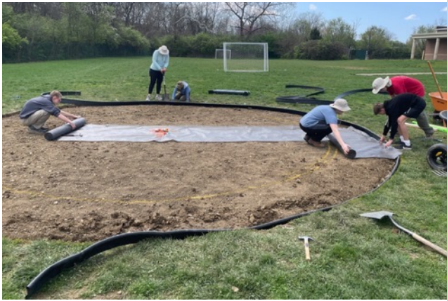
Several scouts started to lay the landscape fabric while several others were finishing up the border
