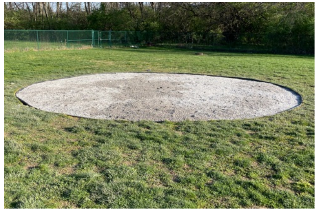
The gravel work is complete
