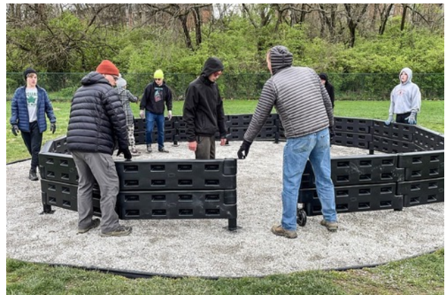
Fine tuning the placement of the wall
