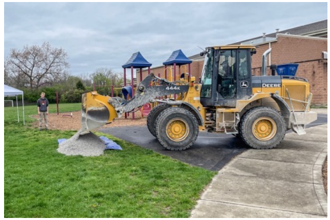
A front loader was used to deliver the gravel
