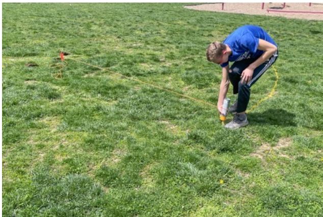
Using a string attached to the center stake and a can of spray paint, Nathan Young marked the circle where the Gaga pit was to be located
