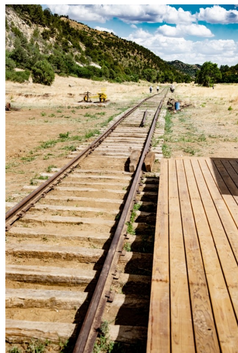
View down the rail line being built at Metcalf Station
