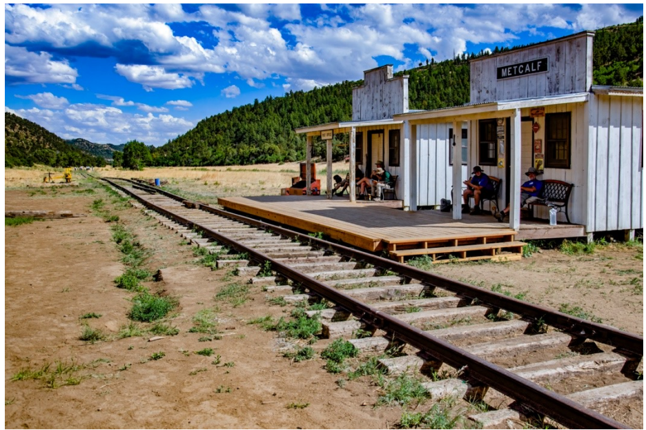
A view of the rail line through the canyon at Metcalf Station
