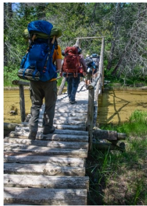
Bridge over Beaver Creek
