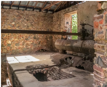
The steam boiler that was added after slave labor was abolished
