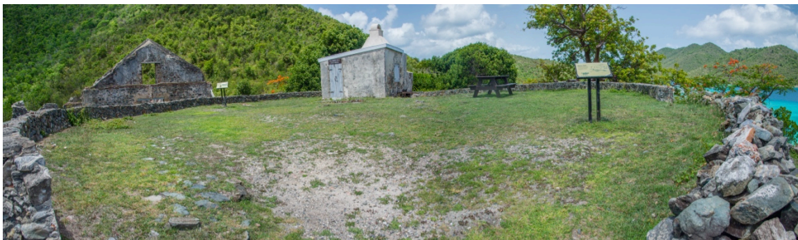
When the wind died, oxen, mules, or horses provided the power for the factory. The animals, harnessed to a drive shaft, would walk in circles in this area to turn the machinery.
