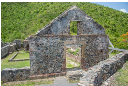
Wall of the main factory room
