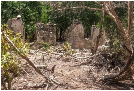
Foundation for an out-building
