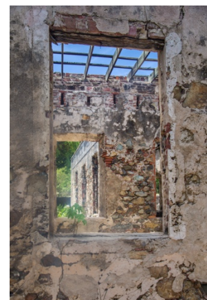
Looking through several rooms
