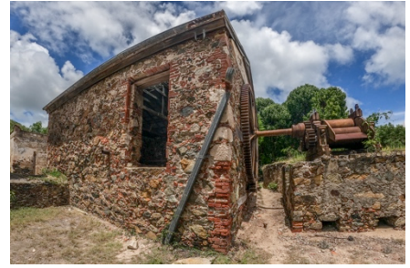
Outside view of one of the mill buildings
