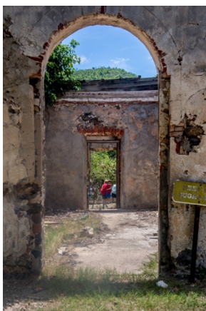
Looking through several rooms
