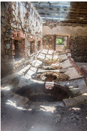
The cane juice was then fed into a series of vats where it was boiled
