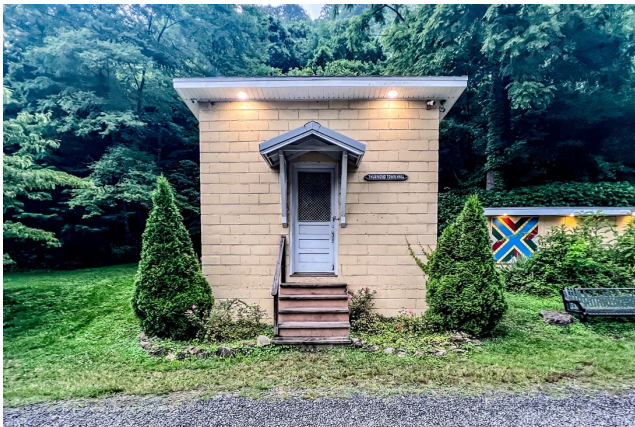
There are still 3 people who live in Thurmond, and this building serves as the town hall.
