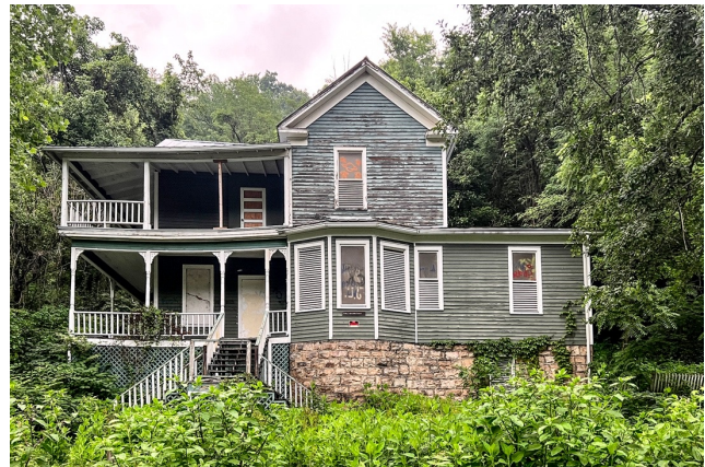
One of the handful of abandoned houses in Thurmond
