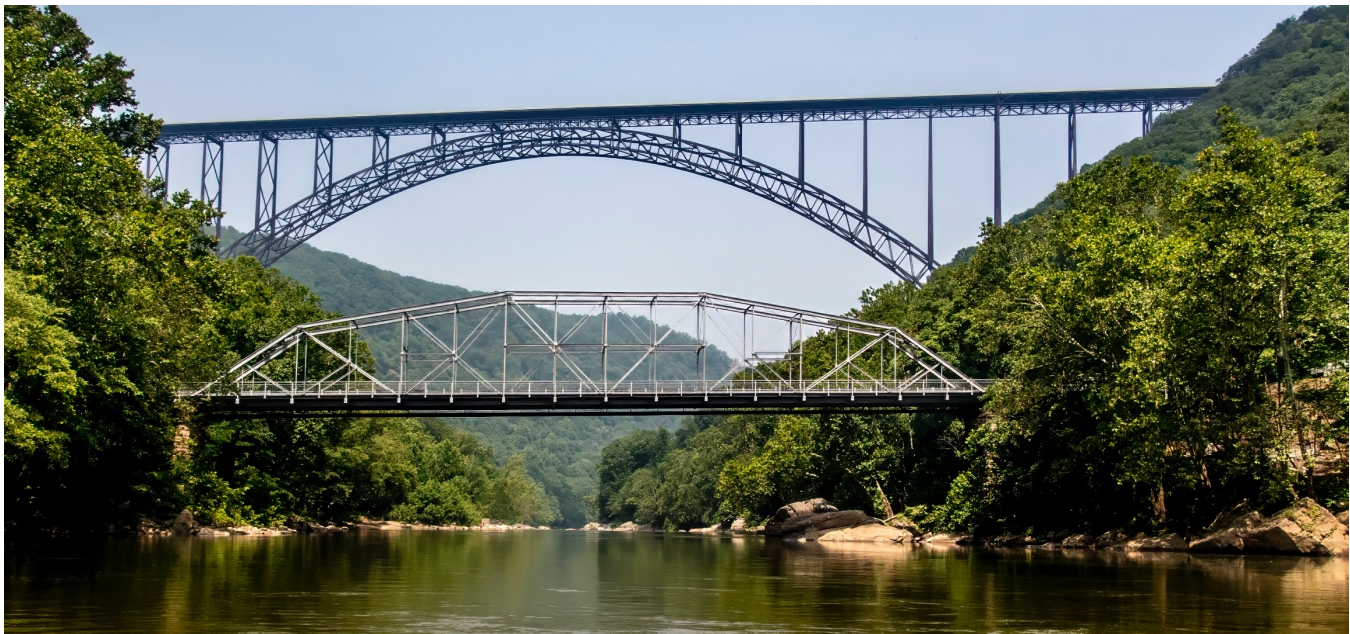
The Fayette Station and New River Gorge Bridges
