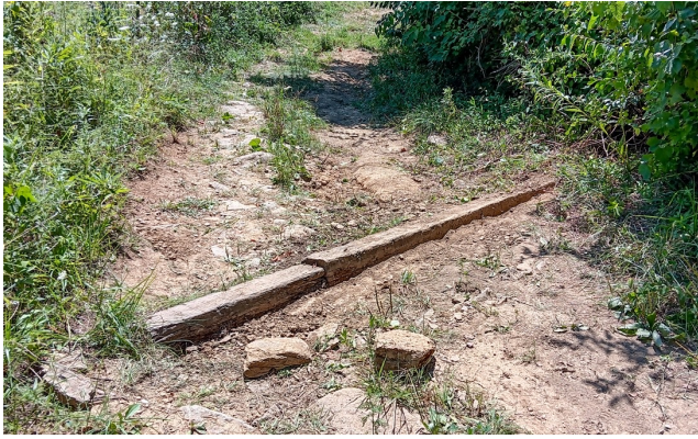
A properly maintained water bar
