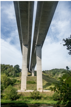
I71 Jeremiah Morrow Bridge over the Little Miami River
