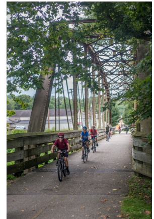
Declan McGrath crossing over Todd's Fork Creek in Morrow, OH
