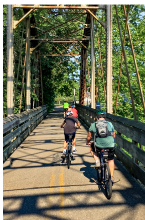
Crossing Todd Fork Creek on the old railroad truss bridge
