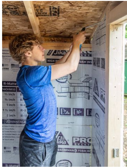
Petey Wilkens using expanding foam to seal the gaps
