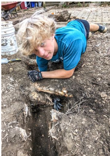
Petey Wilkens digging the trench for the electricity to the shed
