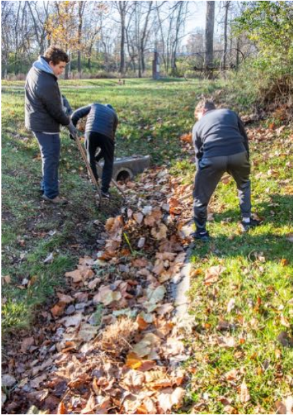
The end of the drainage ravine had a lot of dirt buildup
