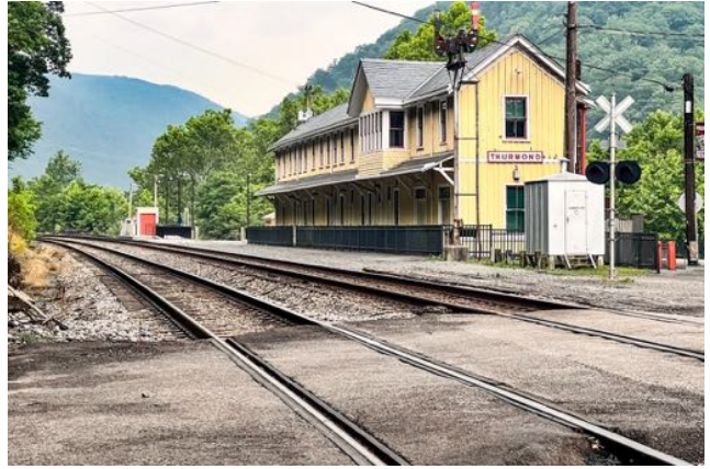
View looking down the tracks to the train station
