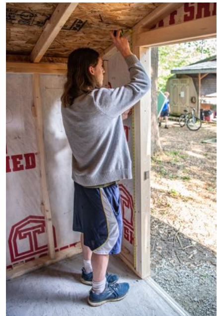
Isaac Lohmueller installing insulation around the door frame
