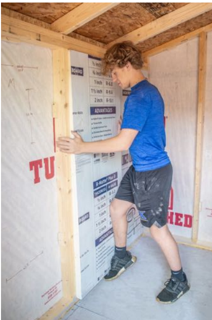
Petey Wilkens installing panels of insulation in the walls
