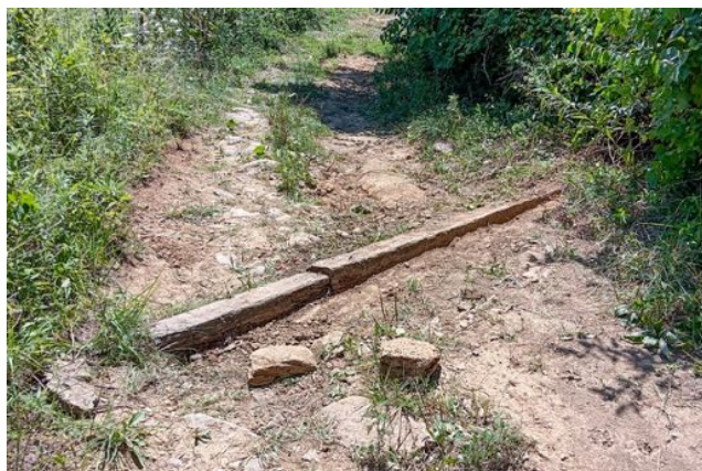
A properly maintained water bar
