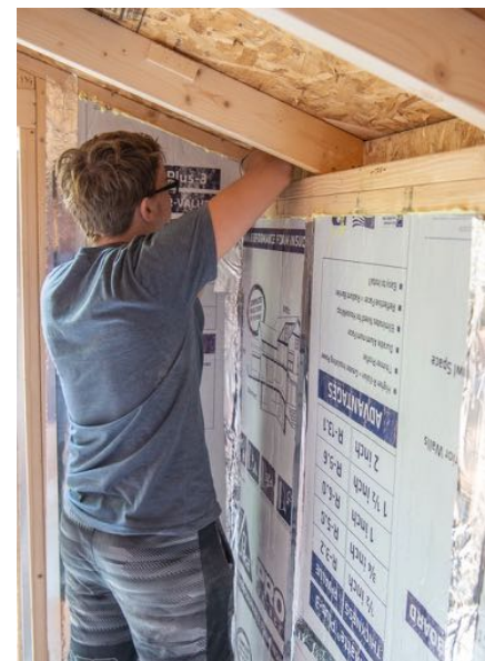
Nathan Hoffman installing small pieces of insulation around the roof
