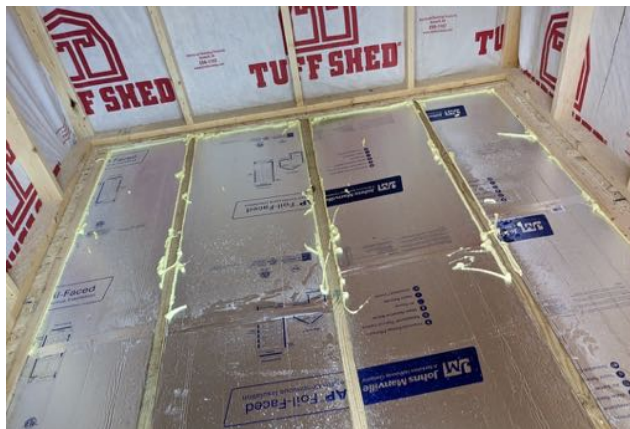
The gaps in the insulation in the floor are being sealed
