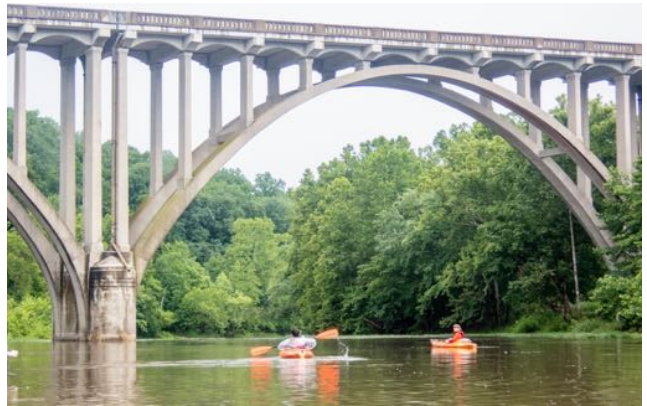
Crossing under the Foster's Bridge
