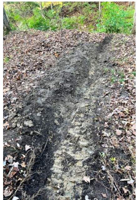
An example of a finished water bar
