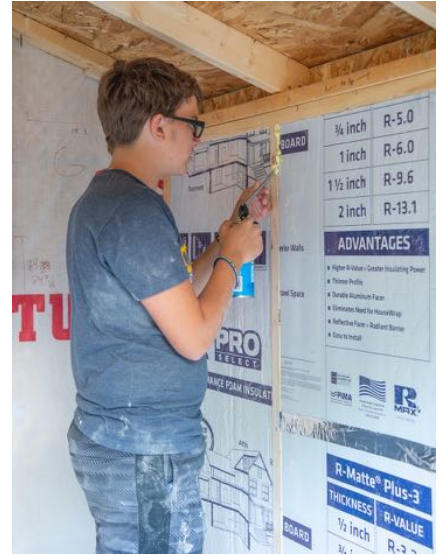
Nathan Hoffman using expanding foam to seal the gaps
